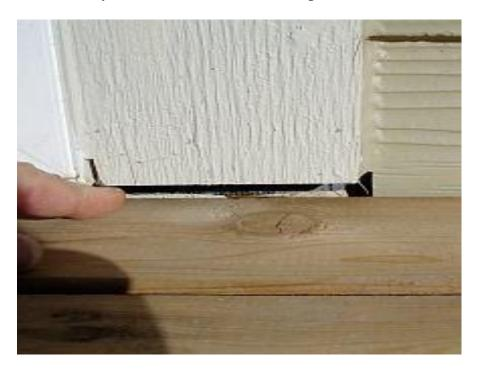
There is no flashing installed at this deck. Consider this: When rain collects on a flat surface (the deck) the water will, inevitably, be routed against the exterior wall. That may lead to seepage of water into the wall and even related structural damage. It is harder, after the fact, to install a flashing at an existing deck or porch. The irony of it all is that it would have been so easy to put in a proper flashing in the first place. Here is an explanatory photo:
