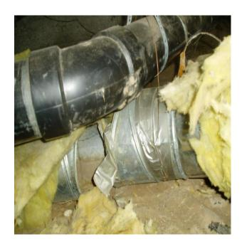
While it might be called "duct tape", duct tape is one of the worst products to use when securing ducts. Home Energy magazine said:
