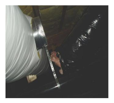
Often, when ducting is disconnected, that is because someone made the original connections, at the joints, with duct tape.
